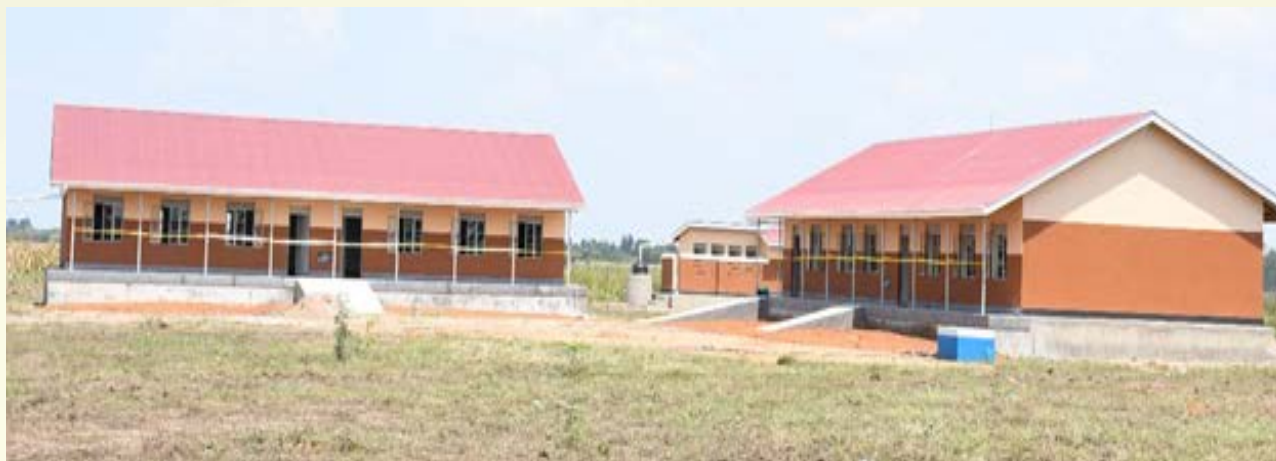
Newly constructed classrooms for Namilyango Primary school at Rwempondo village in Masindi port sub county
