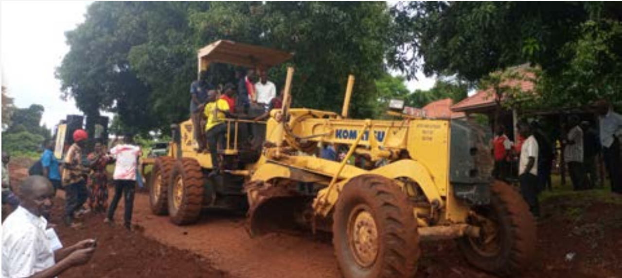
Residents look on as work begins on the upgrade of the Bujwahya-Nyamirima-Kakindo road
