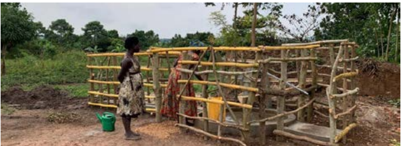
The completed borehole fenced off
